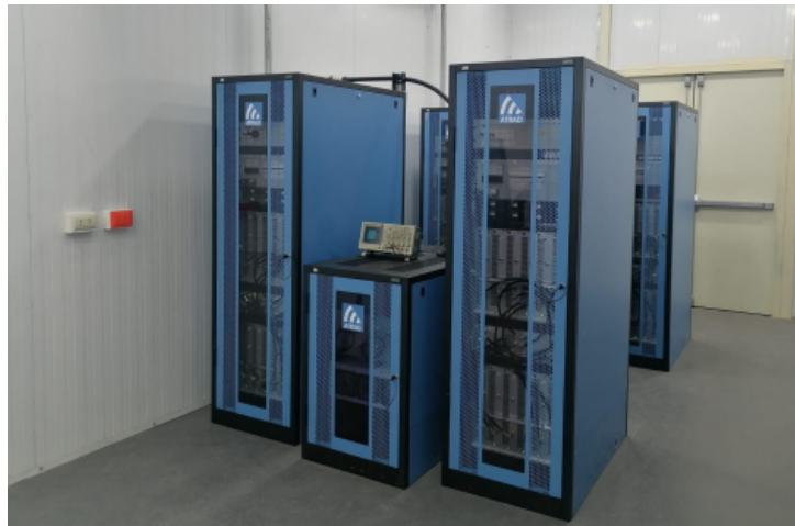
FIGURE 3.4 – The JULIA MP 96 kw solid-state transmitters (KUYENG et al. , 2023).
